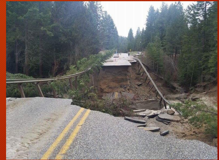
Bridge in Ferry County that washed out during the April 2017 storms. Ferry County Sherriff's office.
